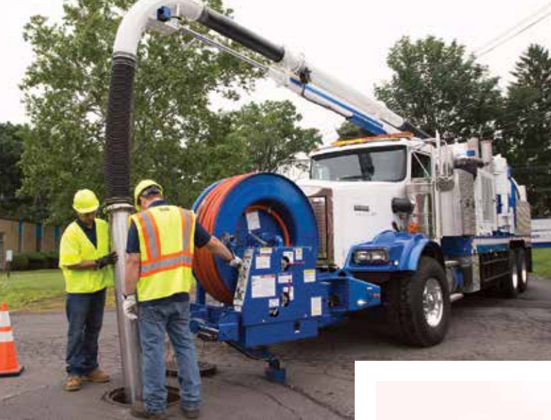
PARSA crew members Steve Grosso (left) and John Malavasi clean out a manhole with their Van-Con truck. The PARSA staff has almost 200 years' combined experience in the wastewater industry.
