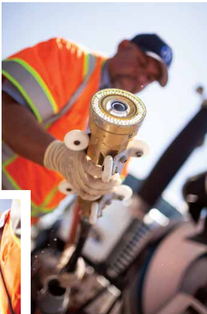
Above: Rene Villalobos prepares the CCTV camera for insertion in a sewer line for a routine inspection. At left: Rene Villalobos (right) works alongside Andie Zetina as they operate Buena Park's CCTV camera.
