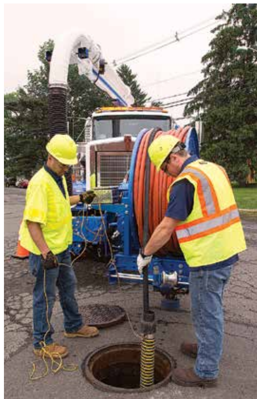
PARSA crew members Steve Grosso (left) and John Malavasi clean out a manhole with their Van-Con truck. The PARSA staff has almost 200 years' combined experience in the wastewater industry.
