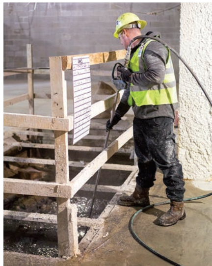
Matt Paules operates the controls on a Vac-Con truck while Joe Hatton uses a spray gun to clean a pit.
