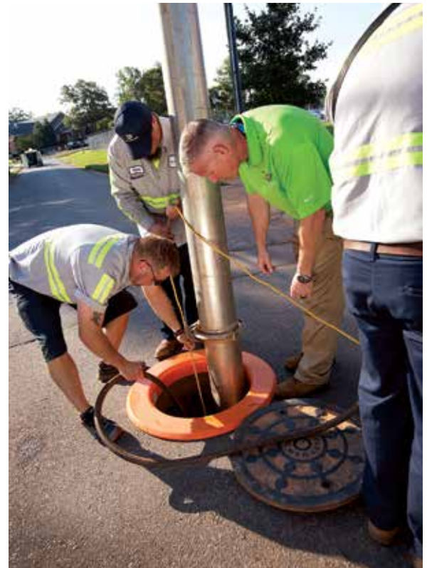
CLOCKWISE FROM LEFT: The Fort Mills Utilities team includes (from left) crewman operator Mike Evans, Utility Operations Superintendent Ben Wright, and crewman operator Travis Blackwelder; Ben Wright (right) checks progress while the crew vacuums debris from the sewer main; Wright ties off a rope connected to the lead on the jetting hose.
