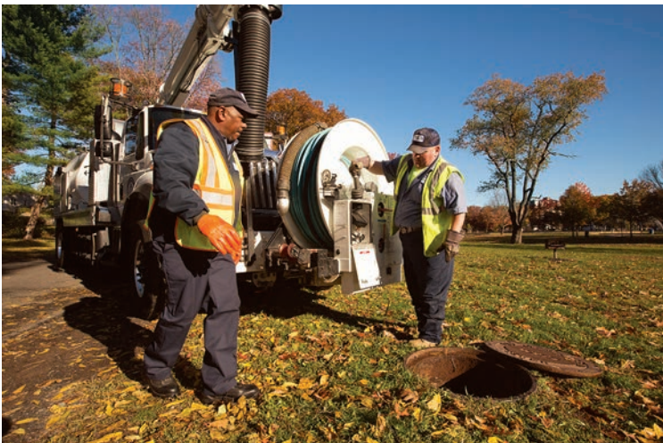
Sewer technicians Steve Bouie (left) and Joseph Mistretta set up their Vac-Con and feed the jetter hose down the manhole to begin cleaning a sewer line.
