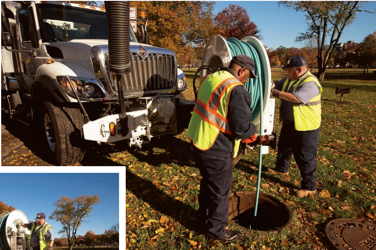
Sewer technicians Steve Bouie (left) and Joseph Mistretta set up their Vac-Con and feed the jetter hose down the manhole to begin cleaning a sewer line.
